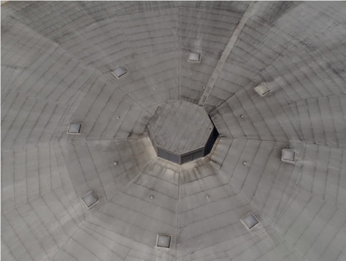
Roof image (left) taken by drone with a digital camera and (right) taken with infrared thermal imaging camera. The white/light yellow colors indicate warmer temperatures, and the black/purple areas indicate cooler temperatures. The vents on the sides of the central structure are cooling the structure (as they are designed to do). The skylights dotted around the central structure are also cooler than the surrounding dome material.
